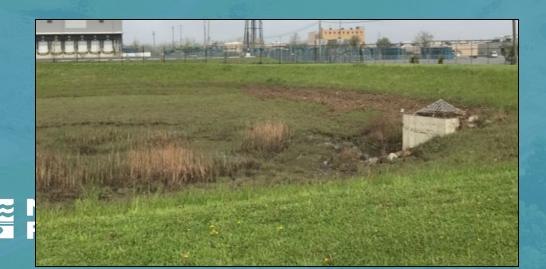
Flow of water is slowed through basin. Basin is dry is dry weather.
