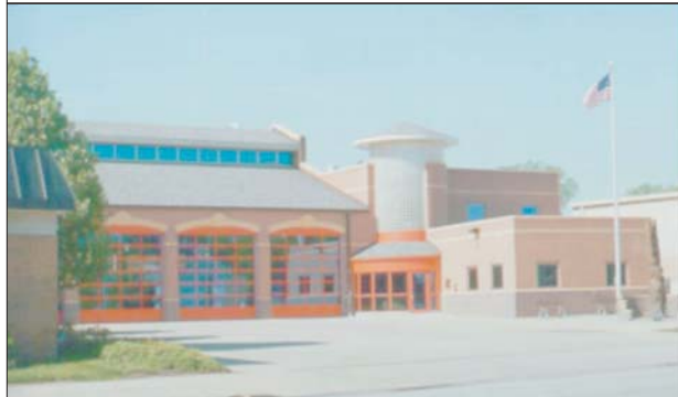
Fire Station Number 1 14601 Madison Avenue Lakewood, Ohio
